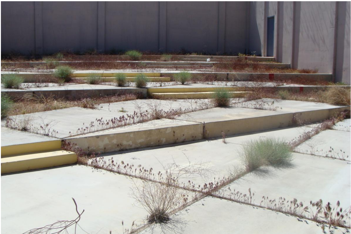
Administration/ Visitation - Building #0176 Description: View of Visitation patio area.
