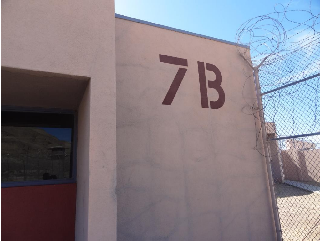
Housing Unit 7 - Building #0187 Description: Exterior of the building.
