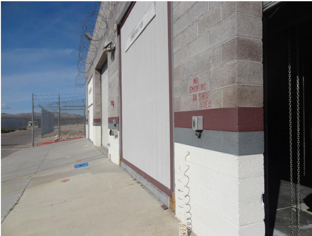
Auto Maintenance Shop/ Warehouse - Building #0192 Description: Exterior of the building.
