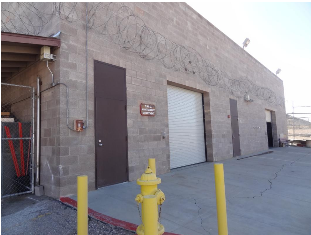
Maintenance Shop - Building #0193 Description: Exterior of the building.
