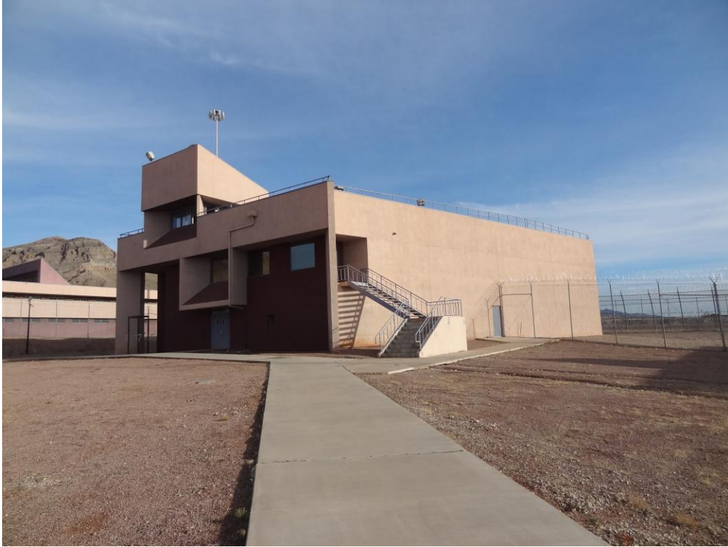
Recreation/ Gym - Building #0186 Description: Exterior of the building.
