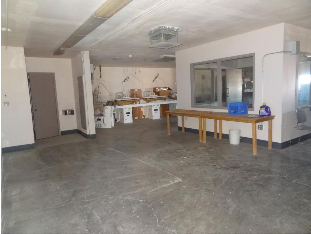
Laundry & Dry Cleaning - Building #0191 Description: Interior of the building.
