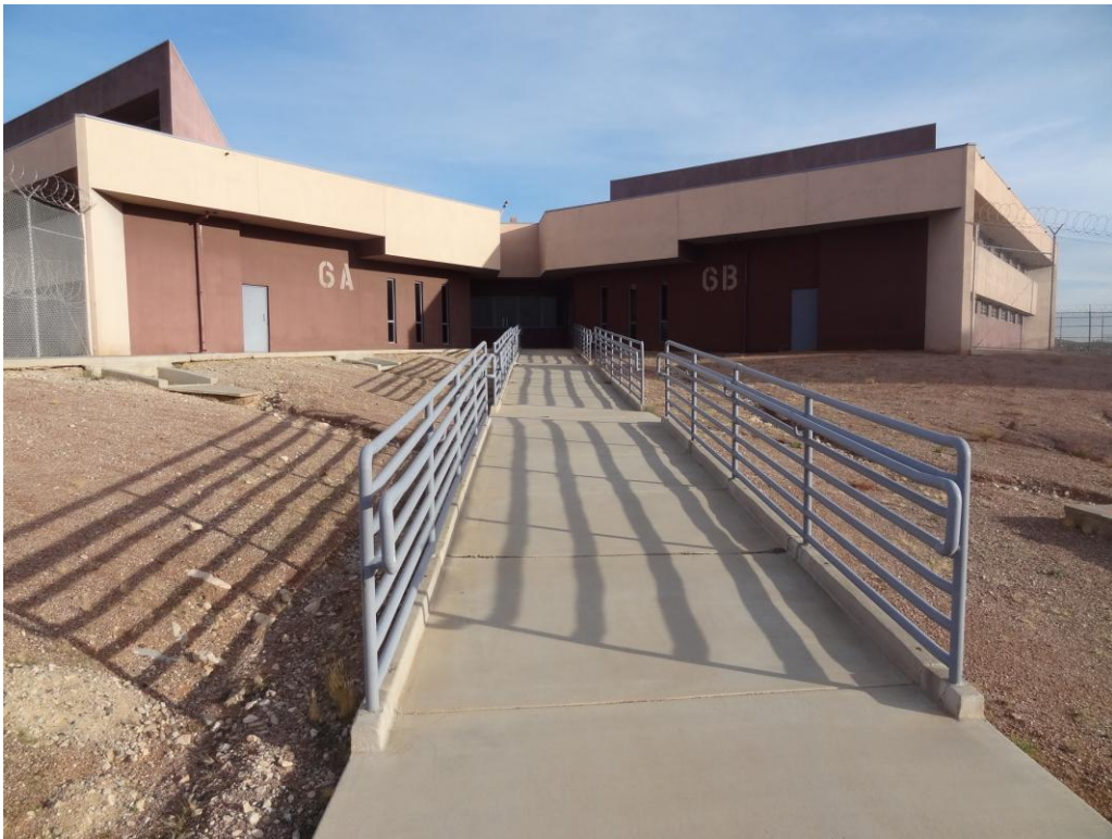
Housing Unit 6 - Building #0185 Description: Exterior of the building and ADA accessible route.
