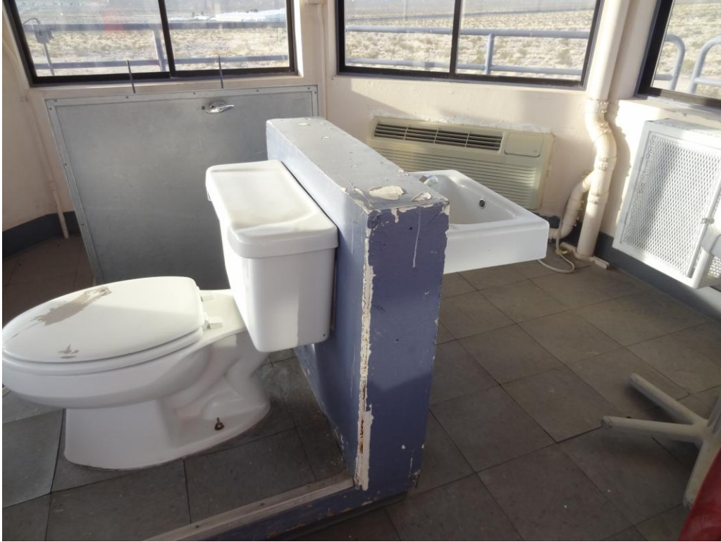
Guard Tower 2 - Building #0195 Description: Interior of the building.
