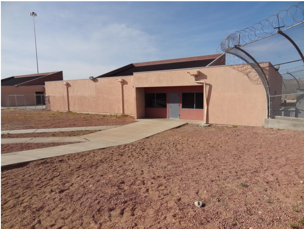
Education A - Building #0178 Description: Exterior of the building.
