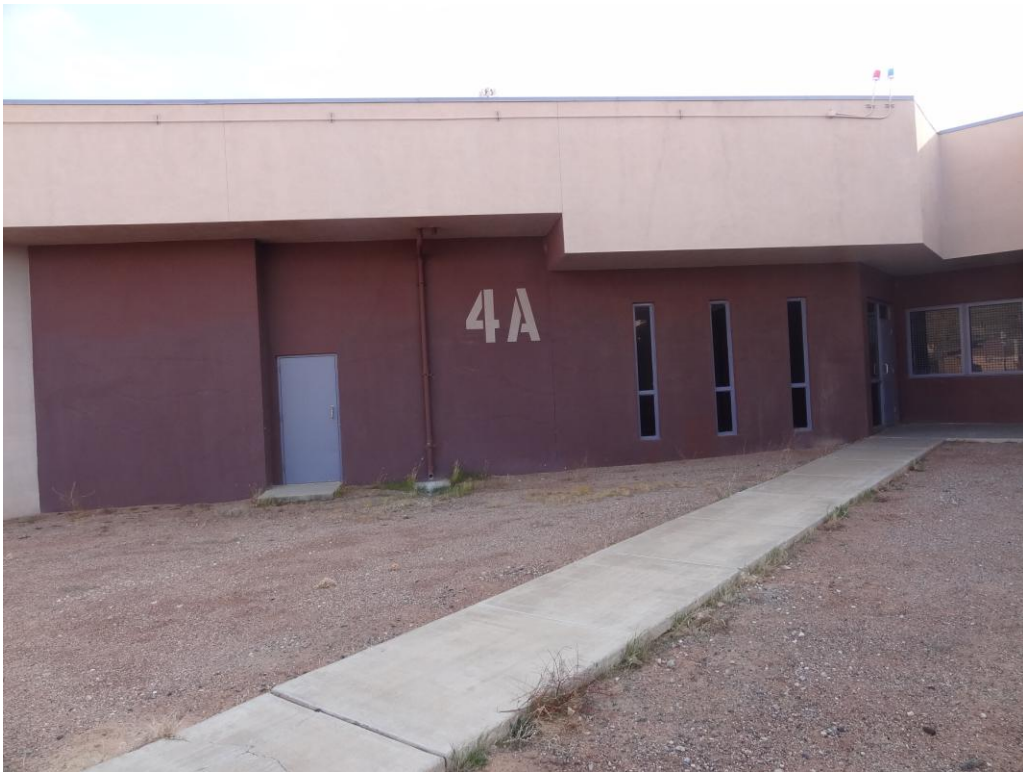
Housing Unit 4 - Building #0183 Description: Exterior of the building.
