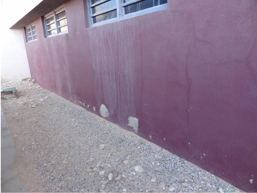
Housing Unit 2 - Building #0181 Description: Exterior of the building.
