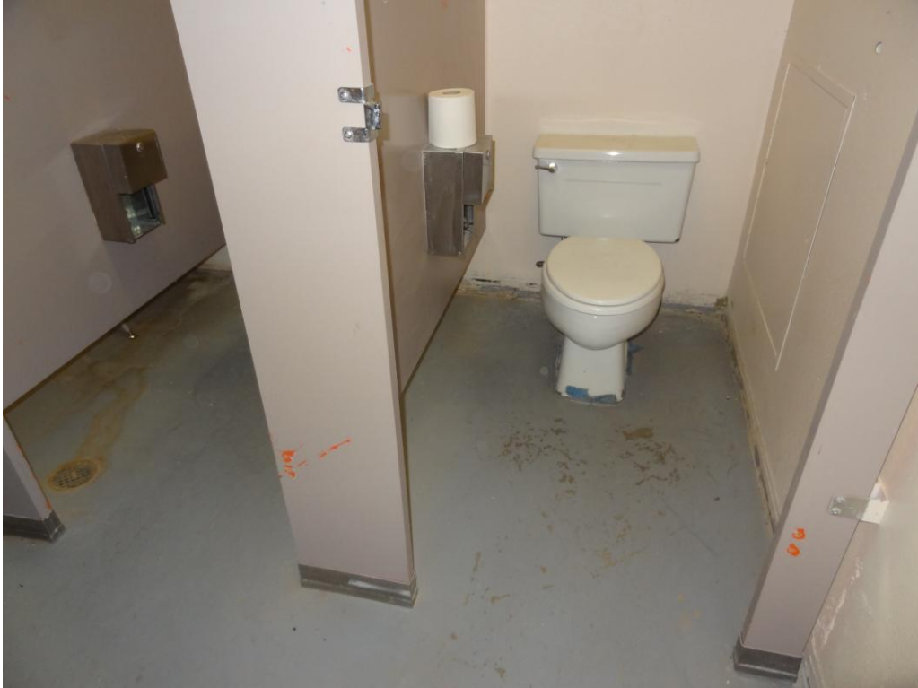
Recreation/ Gym - Building #0186 Description: Typical non-ADA restroom stall.
