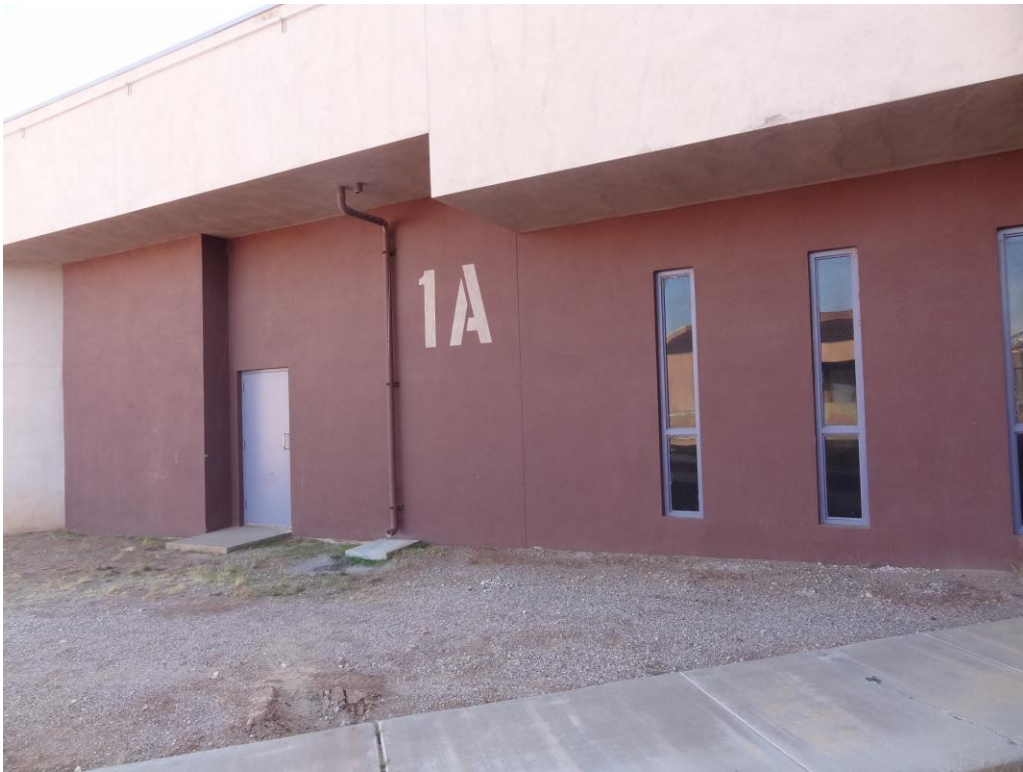
Housing Unit 1 - Building #0180 Description: Exterior of the building.
