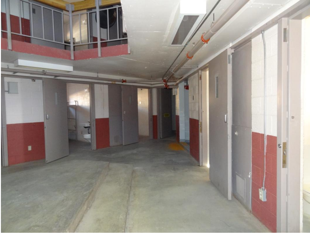
Housing Unit 1 - Building #0180 Description: Interior of the building.
