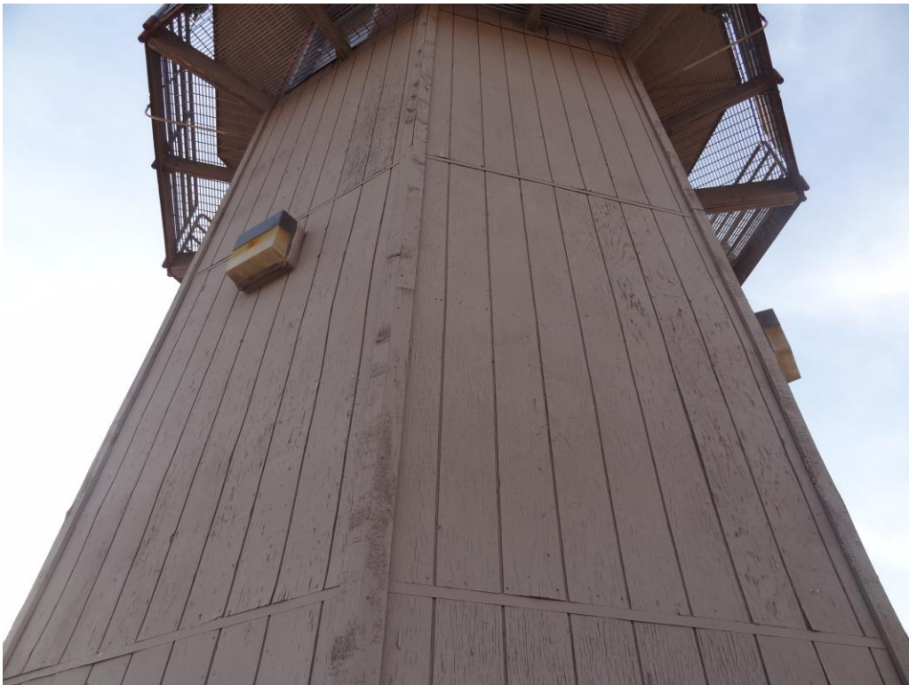
Guard Tower 2 - Building #0195 Description: Exterior of the building.
