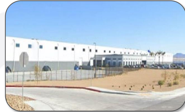
Las Vegas Distribution Center "WDC"
