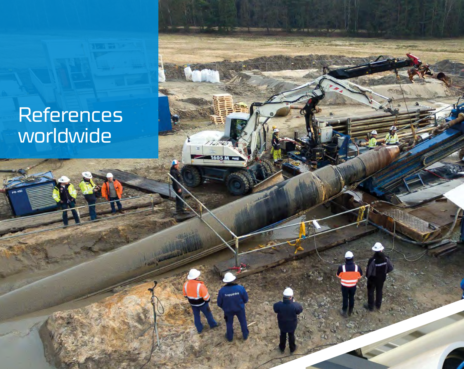
RECORD-BREAKING HDD-INSTALLATION OD 1400 MM
